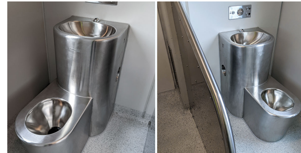
(L-R): Top - A view of Southern Remand Centre build project, view of Britex Stainless Steel Security Privacy Panel, view of Britex Stainless Steel Security Combination Unit and view of Britex Stainless Steel Toilet Security Roll Holder - Rear Fixed.
