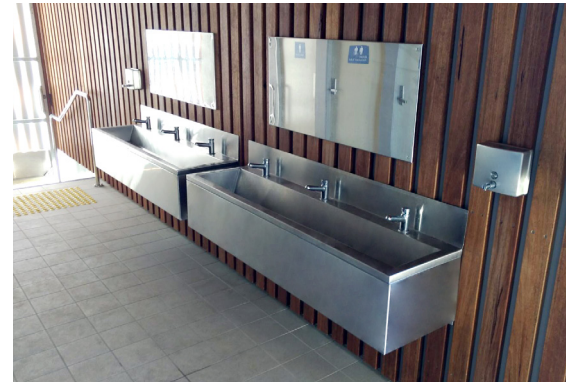
(L-R): Britex S.S. 1500mm No. 4 Pattern Troughs and Britex S.S. Sanistep Urinal.
