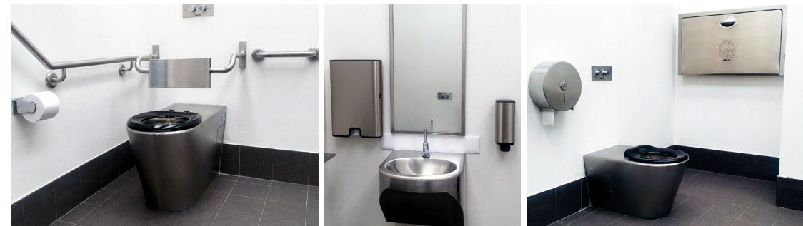
(L-R): Britex S.S. Accessible Hand Wash Basin, Timed Flow Lever Pillar Tap, Britex S.S. In Wall Cistern, Britex S.S. Vandal Resistant Backrest with Combination Rear Rail and RHS Rail with 40 Degree Extension, S.S. Centurion Accessible Toilet Pan with Black Vandal Resistant Closed Front Toilet Seat, Britex S.S. Accessible Hand Wash Basin, Timed Flow Lever Pillar Tap, Britex S.S. Jumbo Roll Toilet Paper Dispenser, Britex S.S. In Wall Cistern, Britex S.S. Centurion Ambulant Toilet Pan with Black Vandal Resistant Closed Front Toilet Seat and Britex S.S. Surface Mounted Baby Changing Station.
