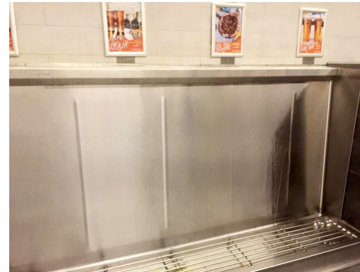
(L-R): Two Britex S.S. Sanistep Urinals at 2700mm
