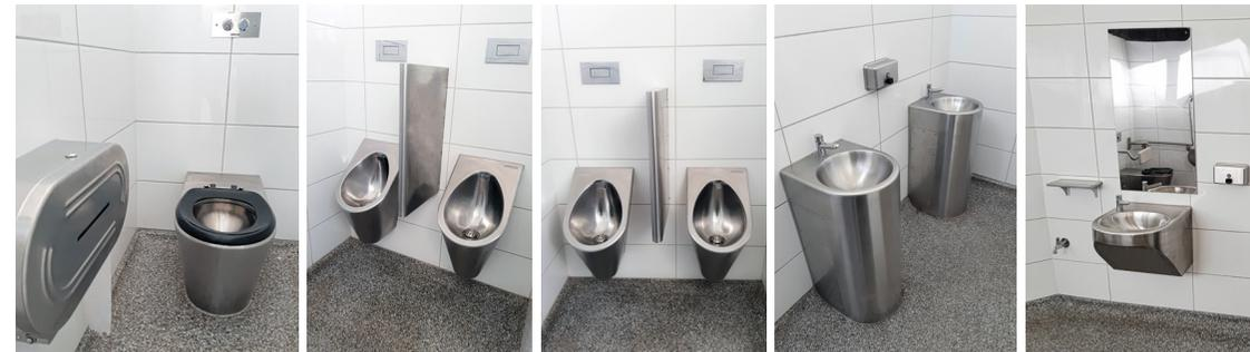
(L-R): Views of Britex Grade Stainless Steel Toilet Cubicle with Stainless Steel Centurion Pan complete with Vandal Resistant Toilet Seat, Britex Stainless Steel Regal Urinal Pods with Britex Stainless Steel Urinal Privacy Panel, Britex Security Pedestal Hand Basins with Access Panel for front access and maintenance, Britex Stainless Steel Accessible Hand Basin.
