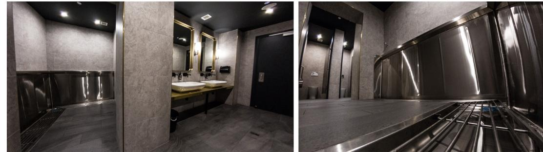
(L-R) The Albion Hotel Mens Bathroom featuring a 4475mm long Britex Stainless Steel Sanistep Urinal in 'L' Shape, delivered and installed on site by the Britex Installation Team.
